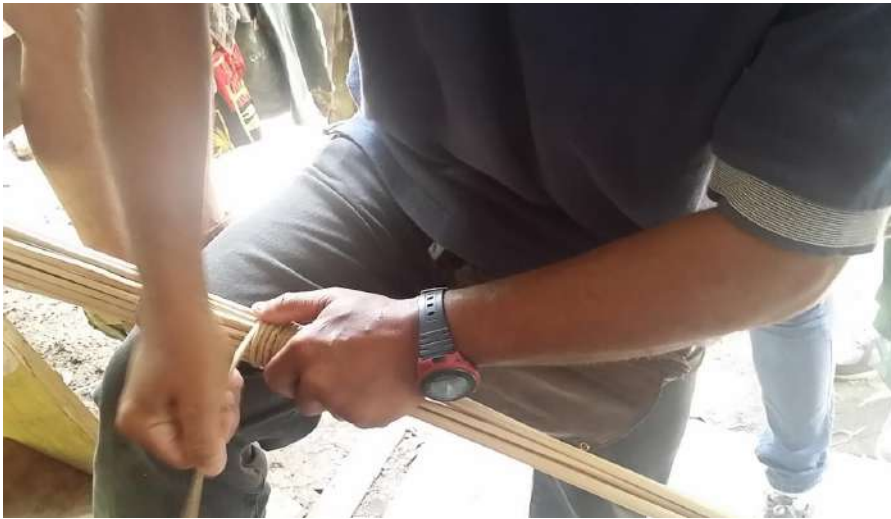
After Mr Raman cut the 5 meter-long bamboo culm into 12 segments, groups of students were asked to round the culms with their craft knives.
