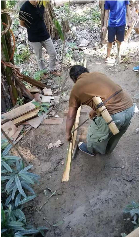
Our bamboo resident in Gombak, Mr Raman, shows how a bamboo culm is split into segments and then prepared in a bundle to form the Pavilion's structure.
